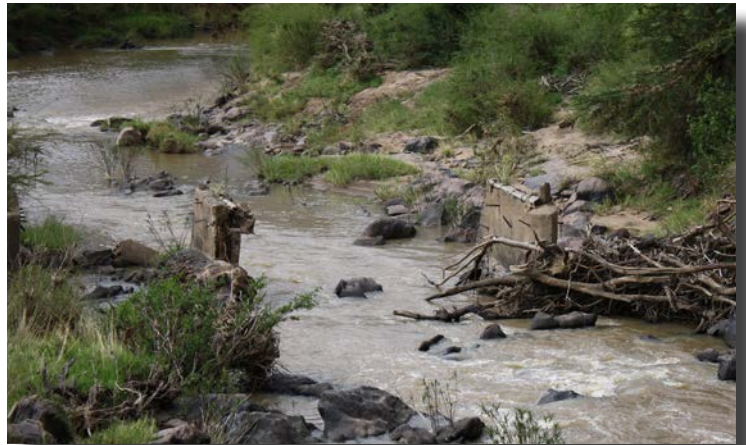
Remains of Princess Hilda's bridge from atop the new bridge. Photo by Laura Budd.
