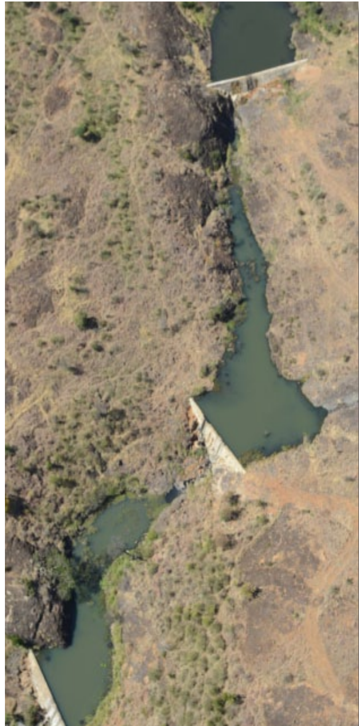
An aerial view of three of the five compartments of Nanja Weirs. Photo by Margaret Kinnaird.
