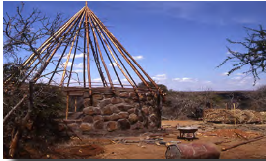
One of the bandas under construction. Photo by Dan Rubenstein.
