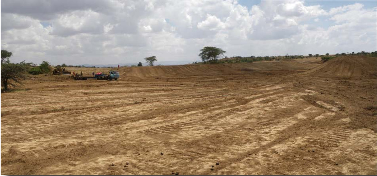
The newly repaired High Dam (above) and Ngaramata Dam (below) await the rains to refill. Photos by Alick Roberts.
